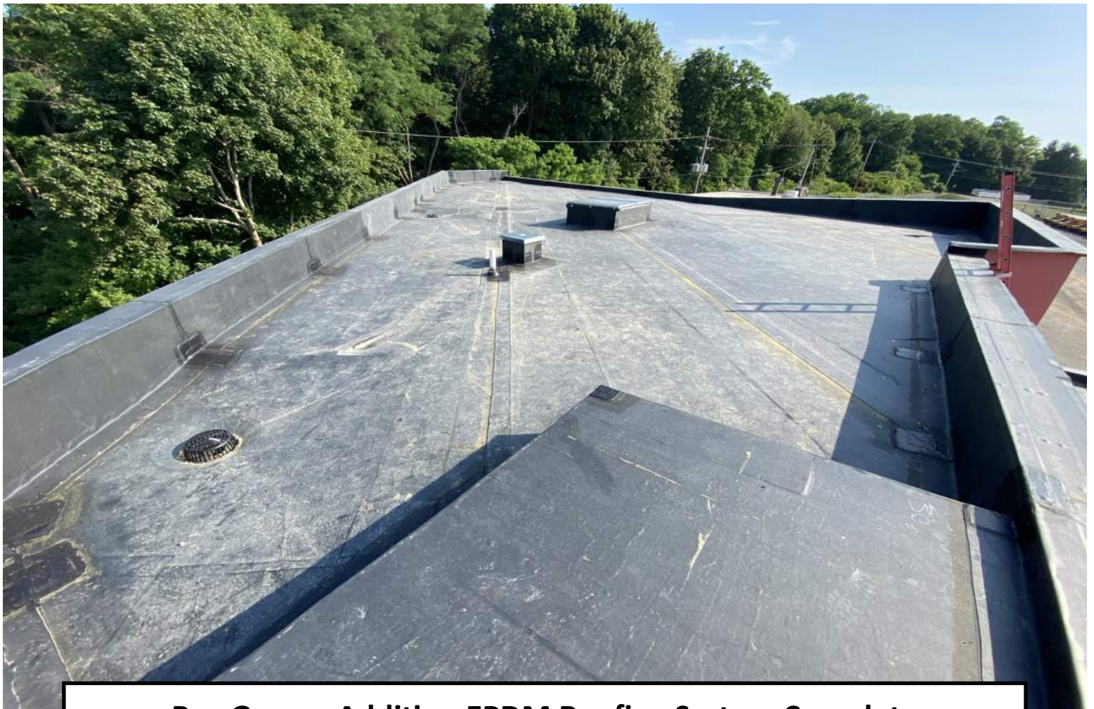
Bus Garage Addition EPDM Roofing System Complete
