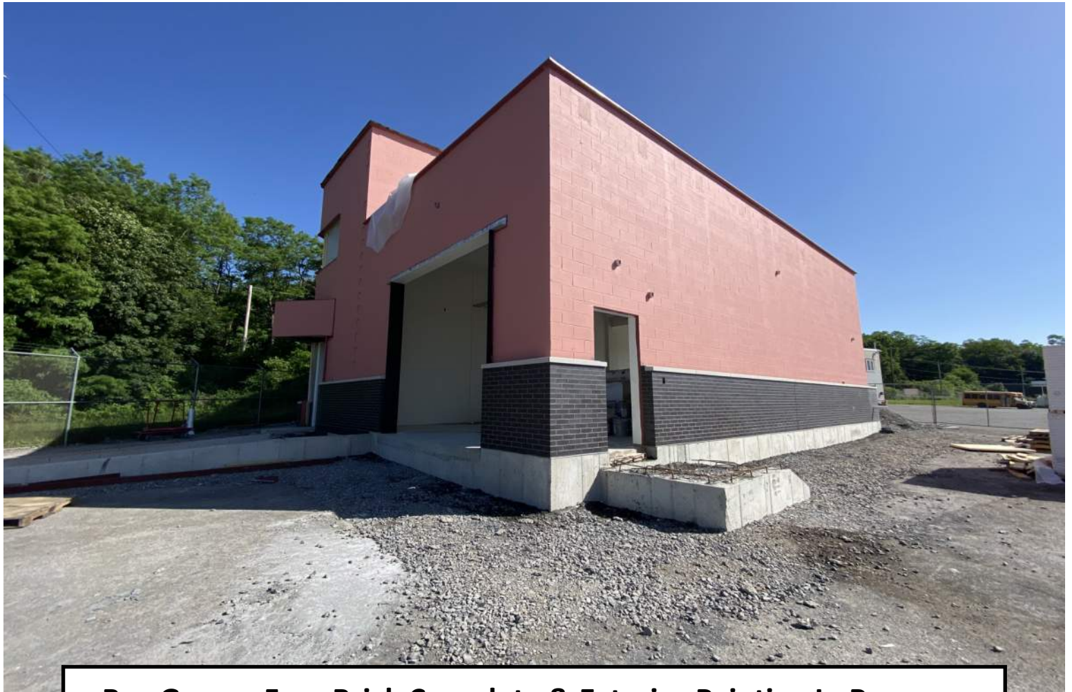
Bus Garage Face Brick Complete & Exterior Painting In Progress
