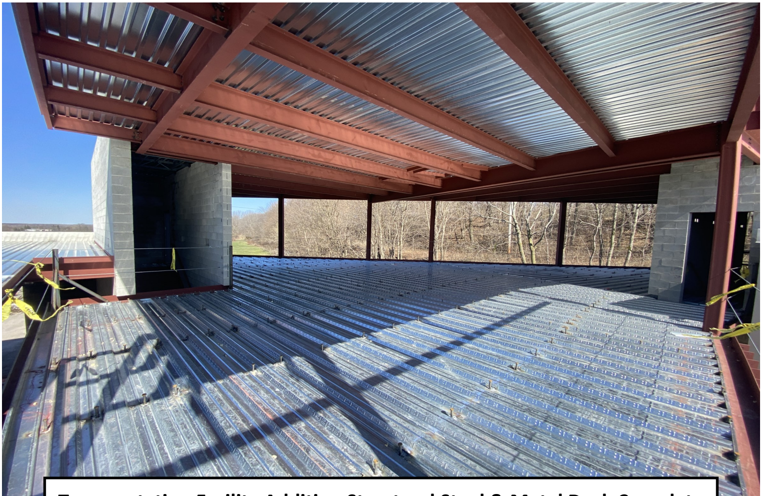
Transportation Facility Addition Structural Steel & Metal Deck Complete
