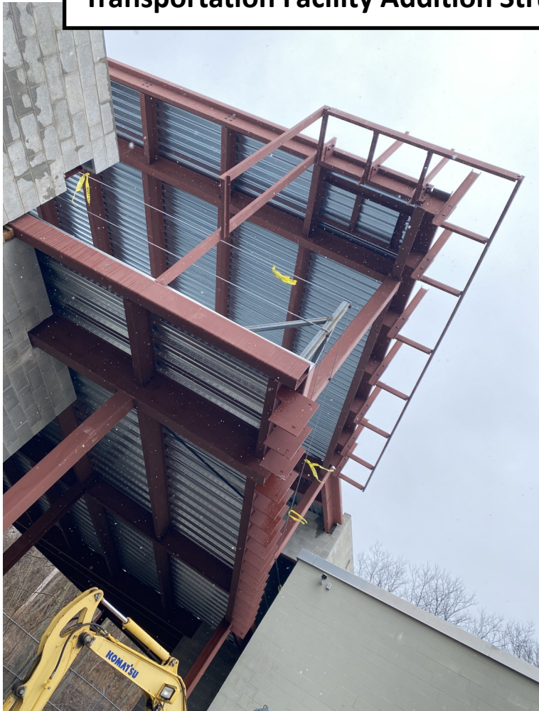
Transportation Facility Addition Structural Steel & Metal Deck Complete
