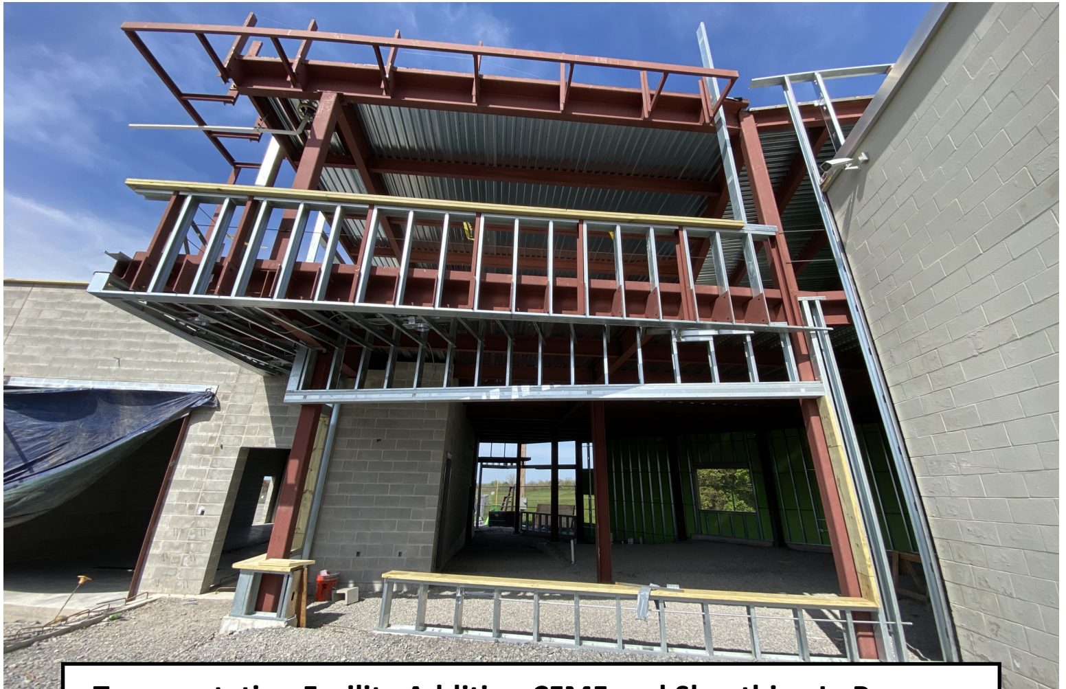
Transportation Facility Addition CFMF and Sheathing In Progress
