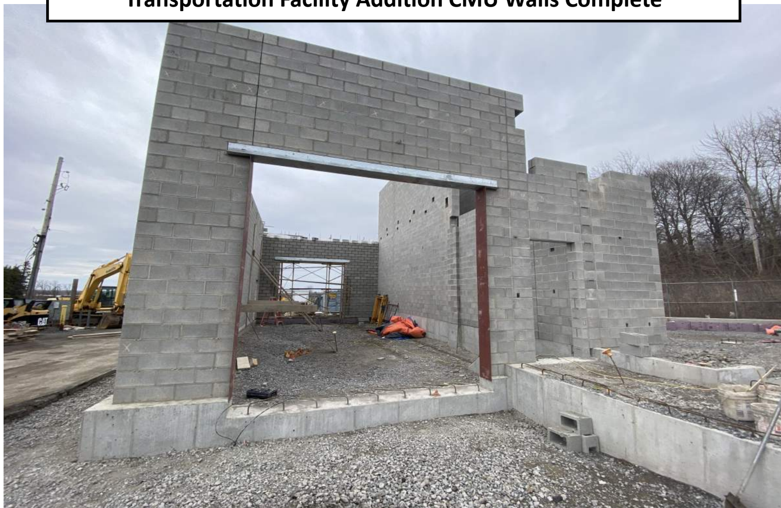
Transportation Facility Addition CMU Walls Complete
