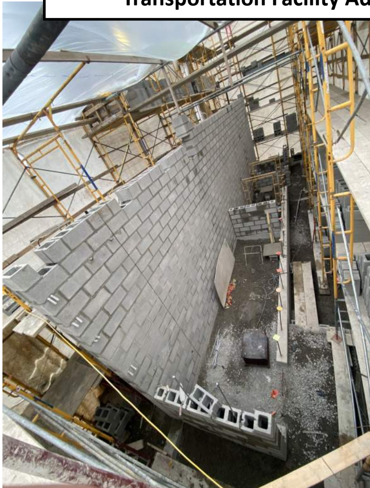
Transportation Facility Addition Masonry In Progress
