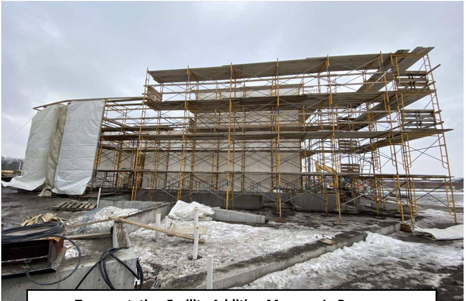
Transportation Facility Addition Masonry In Progress
