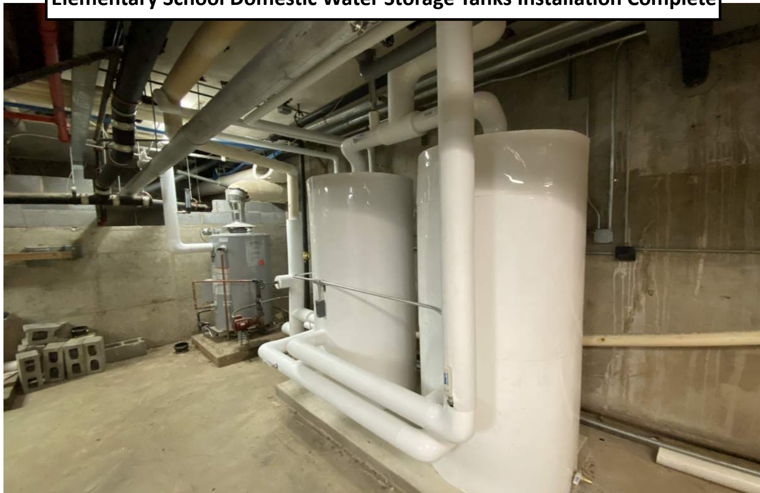
Elementary School Domestic Water Storage Tanks Installation Complete
