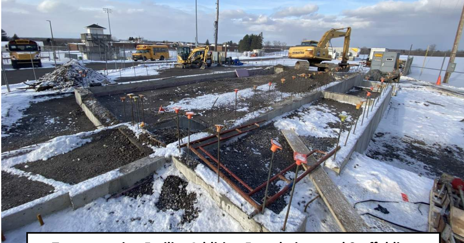
Transportation Facility Addition Foundations and Scaffolding
