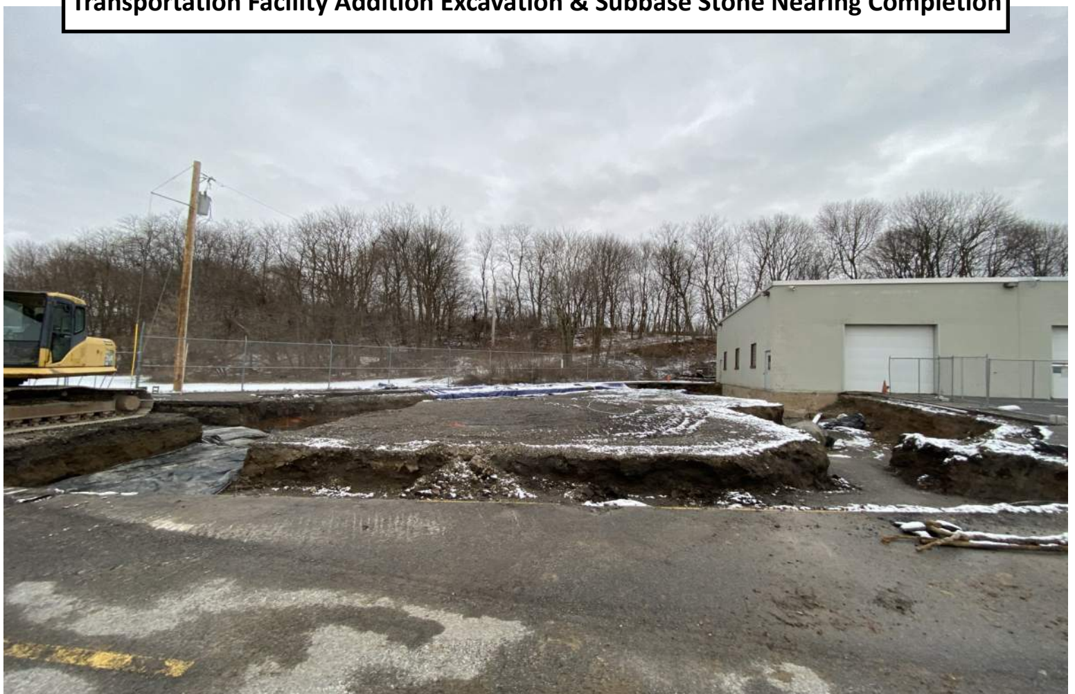
Transportation Facility Addition Excavation & Subbase Stone Nearing Completion
