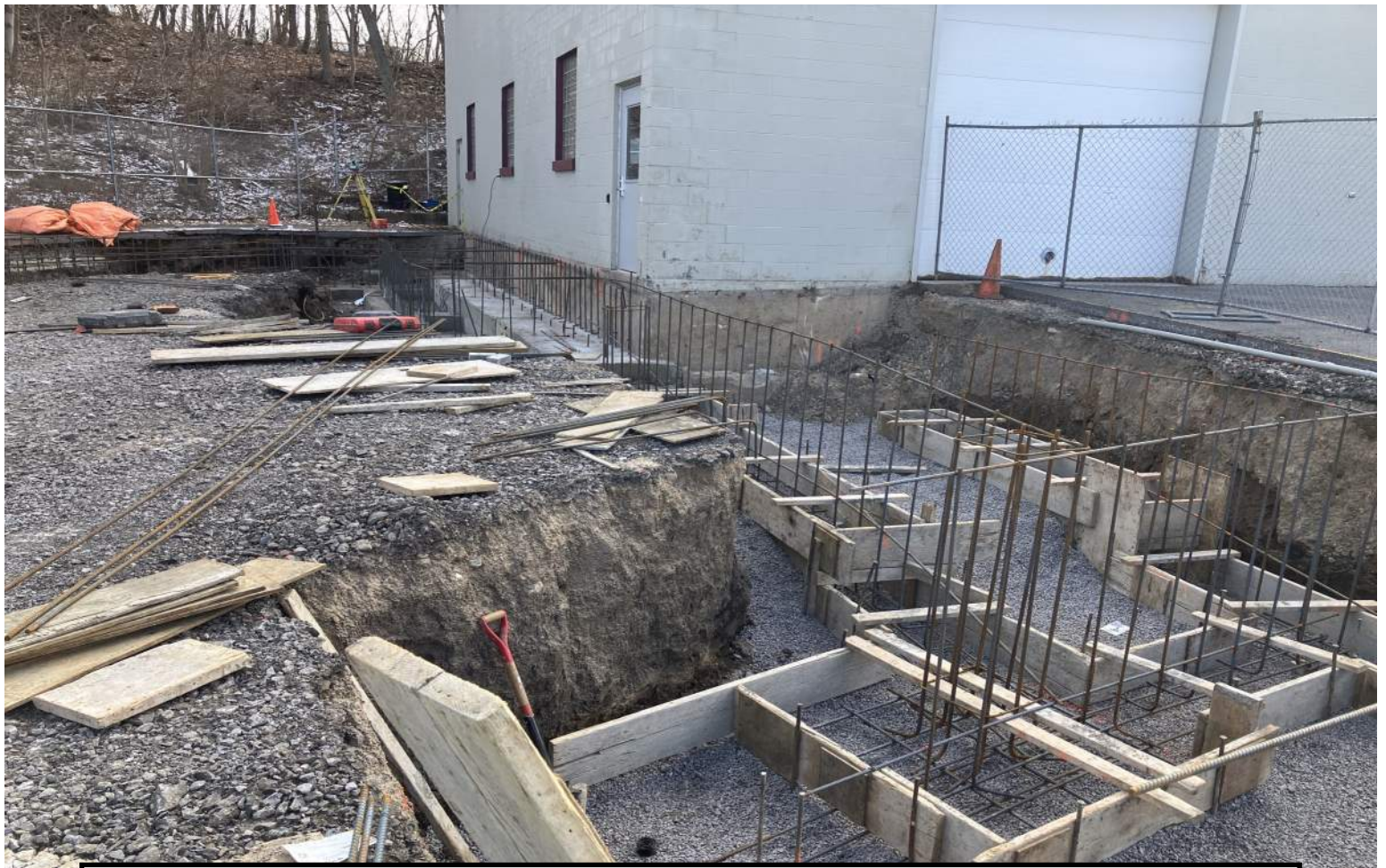
Transportation Facility Addition Foundations In Progress
