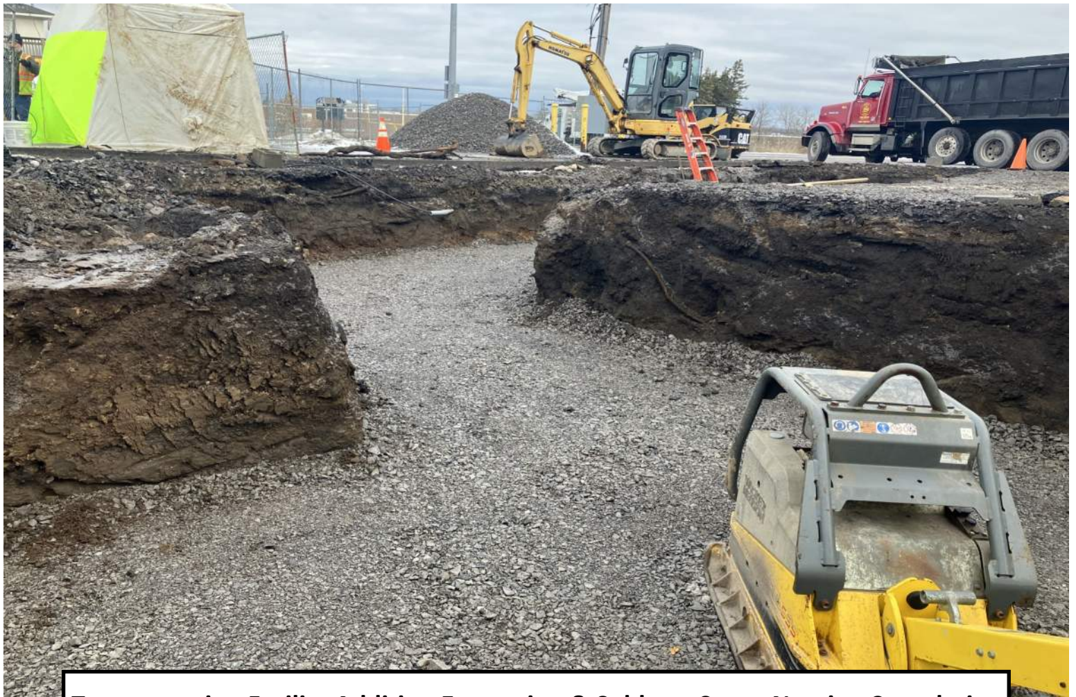
Transportation Facility Addition Excavation & Subbase Stone Nearing Completion
