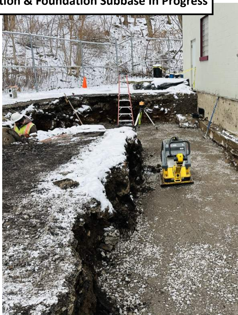
Transportation Facility Addition Excavation & Foundation Subbase In Progress
